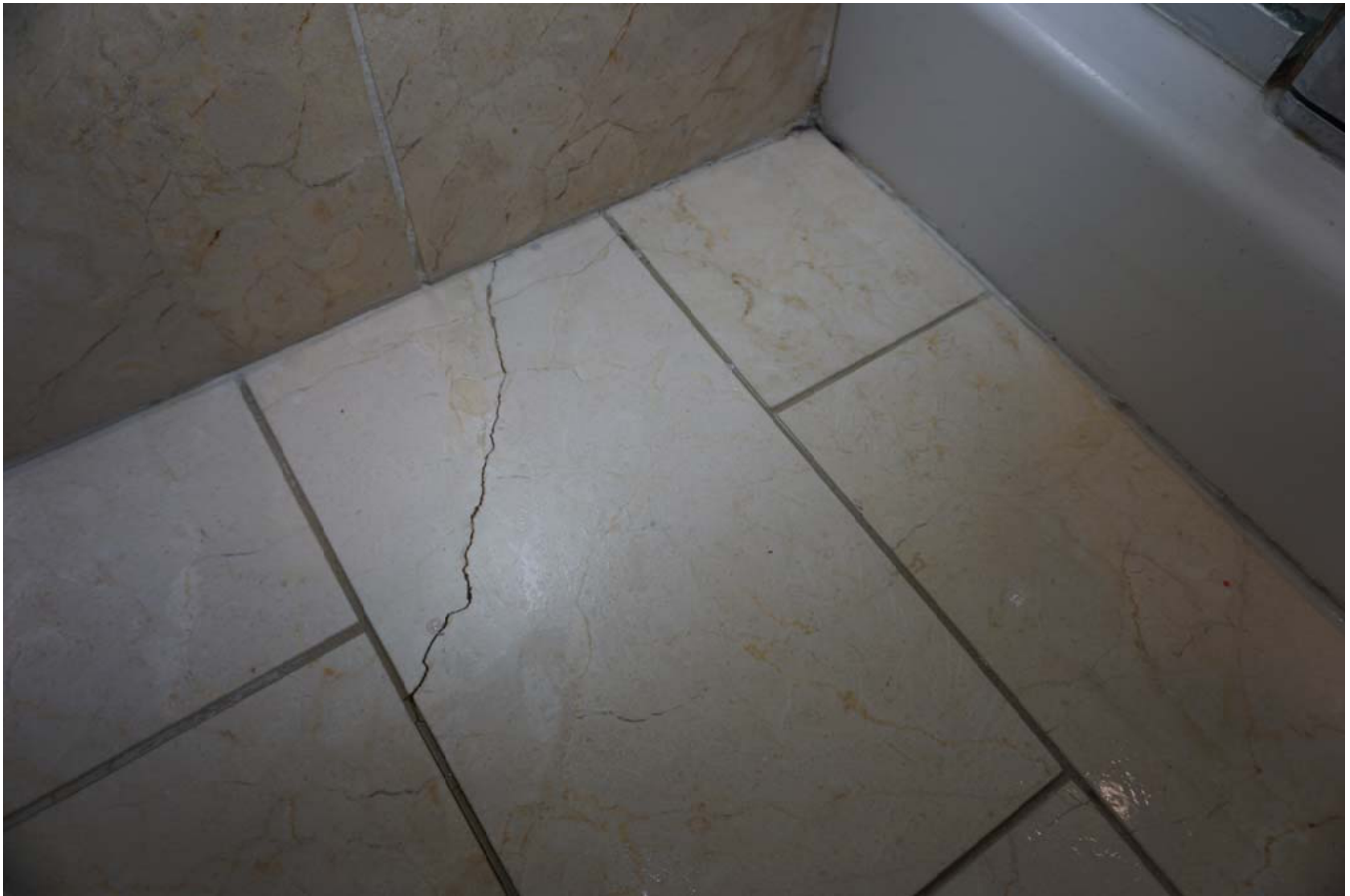
13) Cracked floor tile
