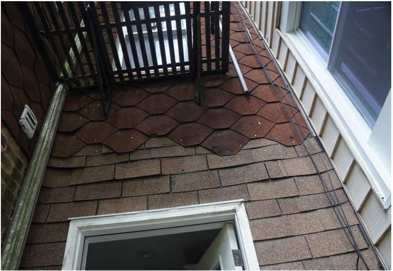
Heavy wear at rear facade
