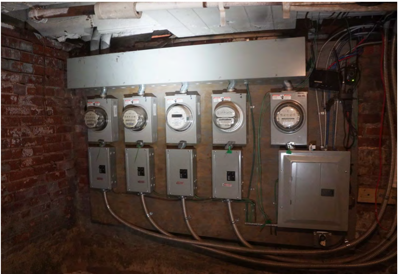
Electric meter & main breakers
