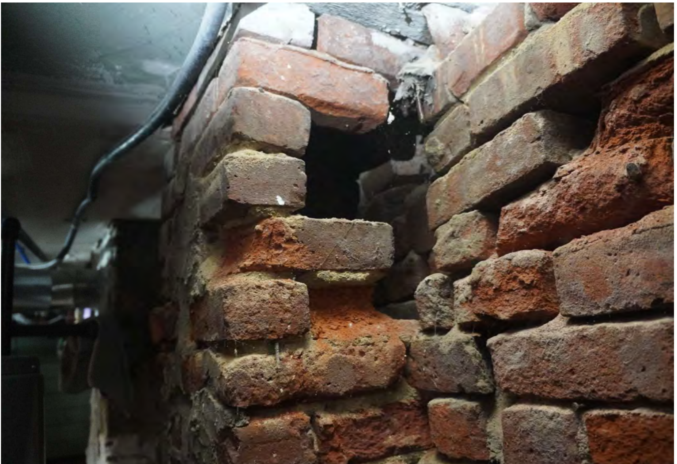
Heavy wear & deterioration at foundation wall
