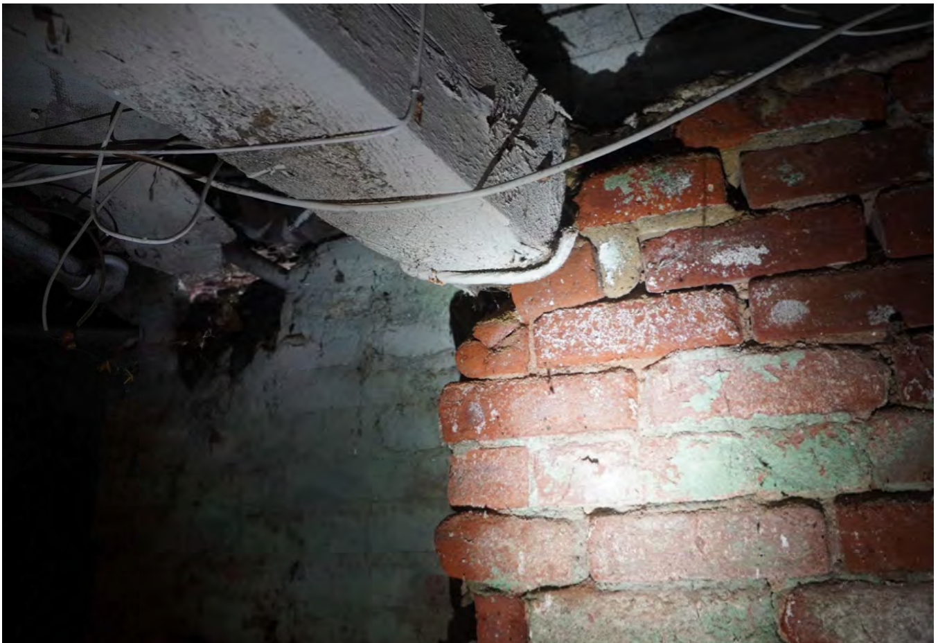
Twisting at main girder
