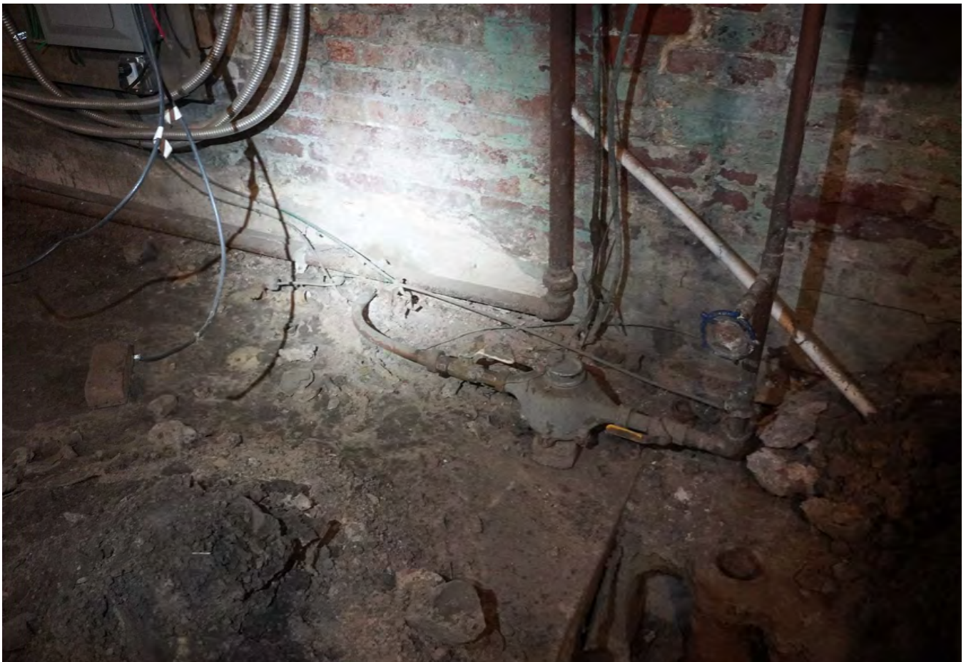
Water meter & main shutoff vale
