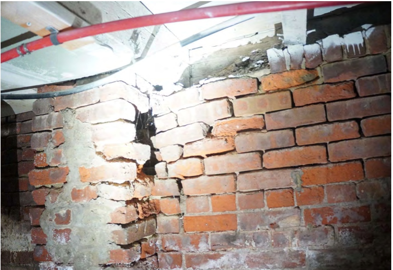
Heavy wear & deterioration at foundation wall
