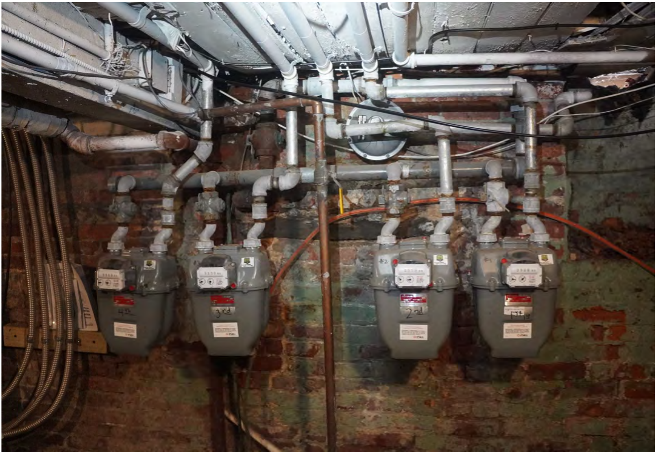
Gas meters & main shutoff valve
