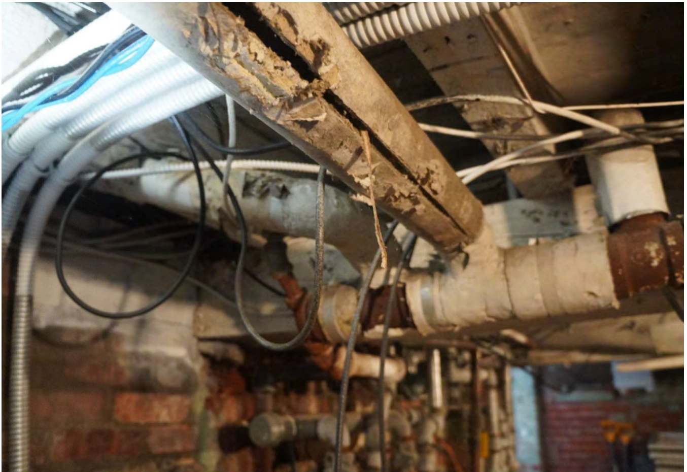
Suspected asbestos containing materials at heating pipes
