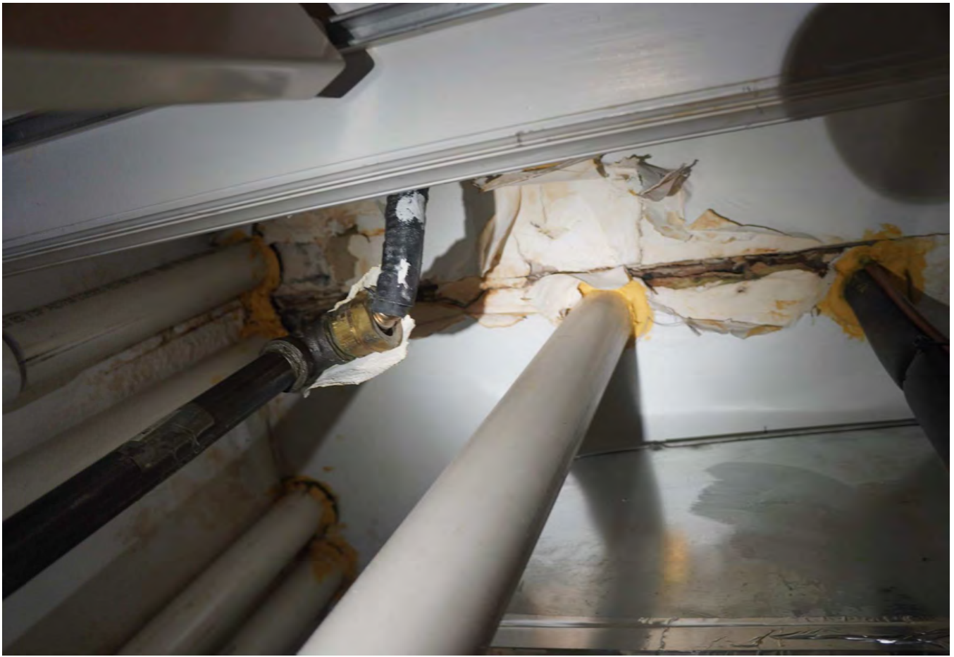
Ceiling moisture damage
