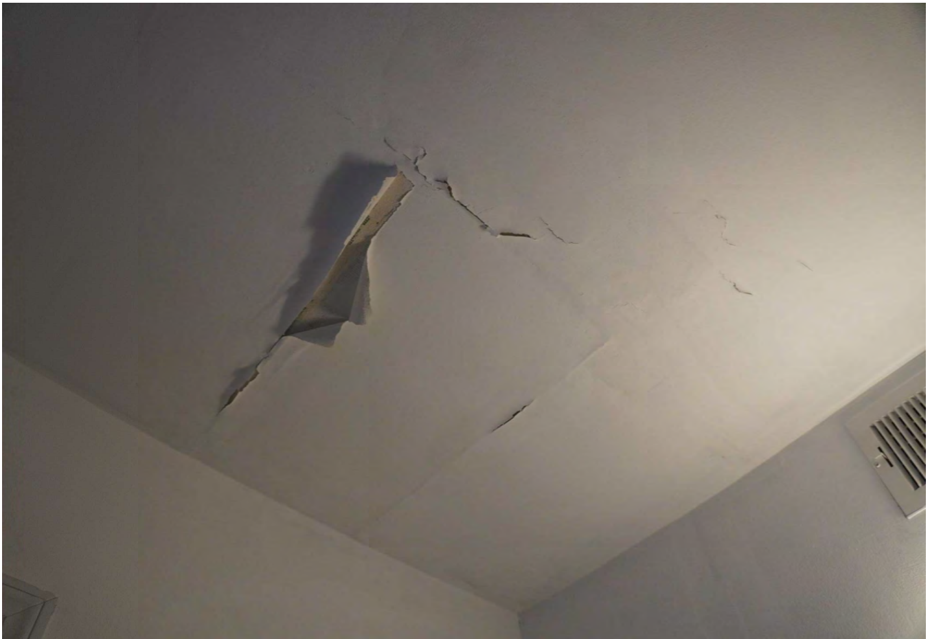
Ceiling moisture damage
