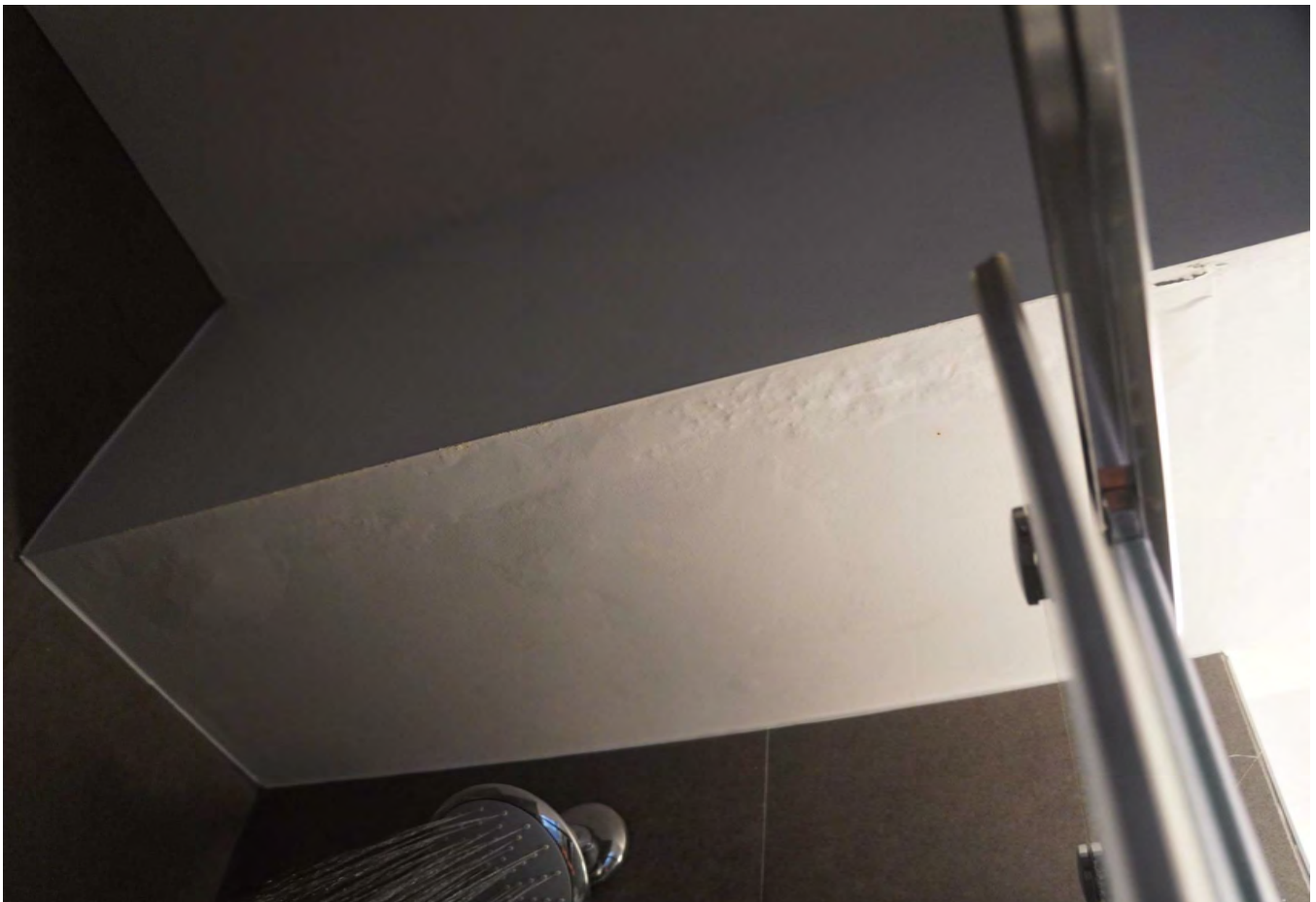
Ceiling moisture damage
